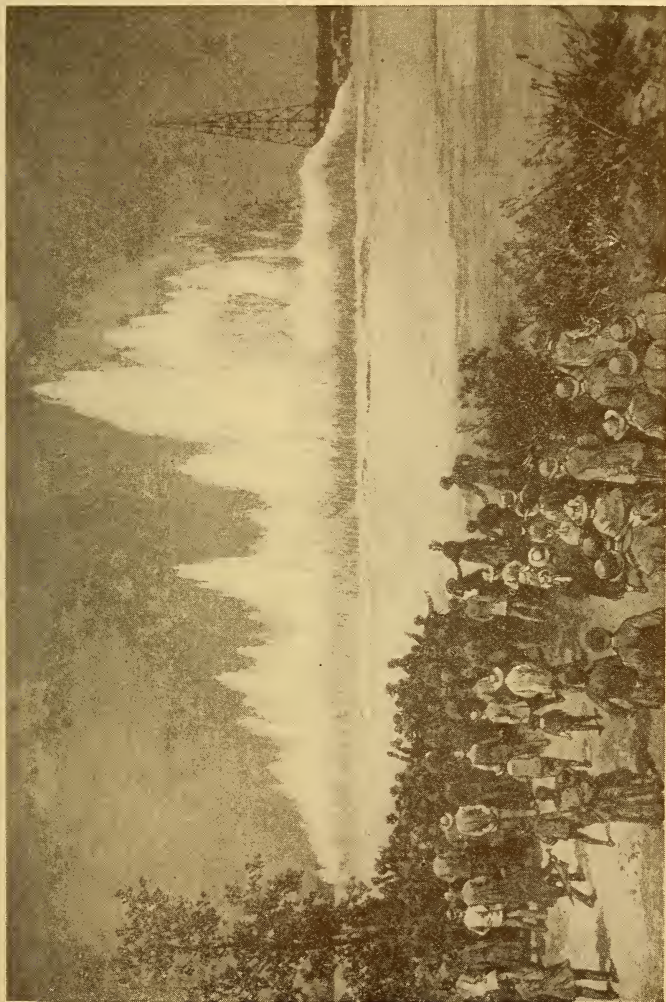
Blowing up of Flood Rock at Hell Gate which removed the last great obstruction to navigation between the East River and the Sound. For its day it was a great engineering feat.
